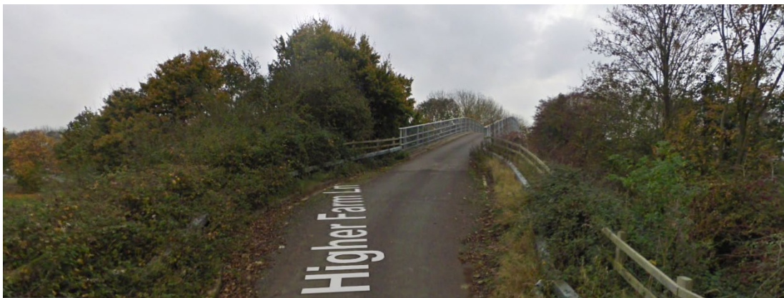
Figure 4: Higher Farm Overbridge from north side approach 42
